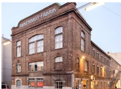
Entrance to Kulturhaus Brotfabrik
